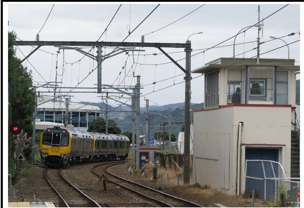
Petone Box number 2 - opened March 1952, closed December 2013.
